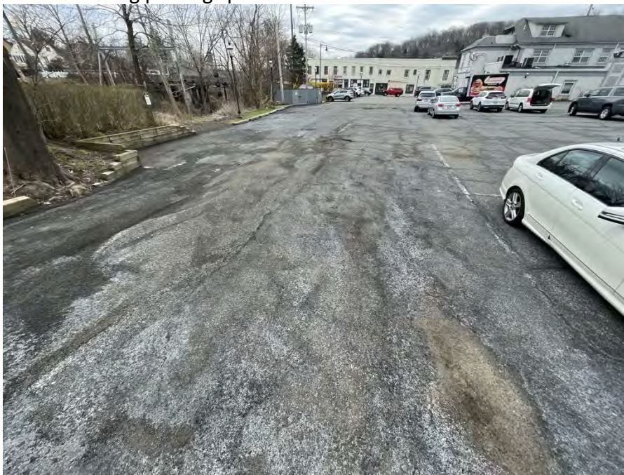
Figure 17: Where the site plan indicates a continuous row of parking to the very rear of lot 1 and 3, several spaces are not marked. This has served to create a de facto, unmarked drive aisle with the elimination of intended parking spaces.
