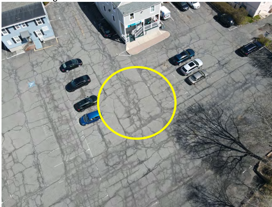
Figure 28: The two-way directional arrows for the drive aisle serving most of the parking on lot 3 are missing. The lack of directional arrows is a condition of faulty arrangement that increases the likelihood of conflict and is detrimental to health and safety.
