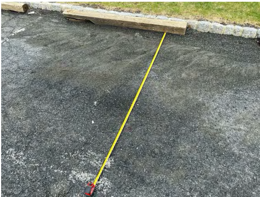
Figure 7: In addition to not being approved on the site plan and being undersized, these parking spaces also reduce the width of the adjacent drive aisle to less than 16 feet across as shown in Figure 8.
