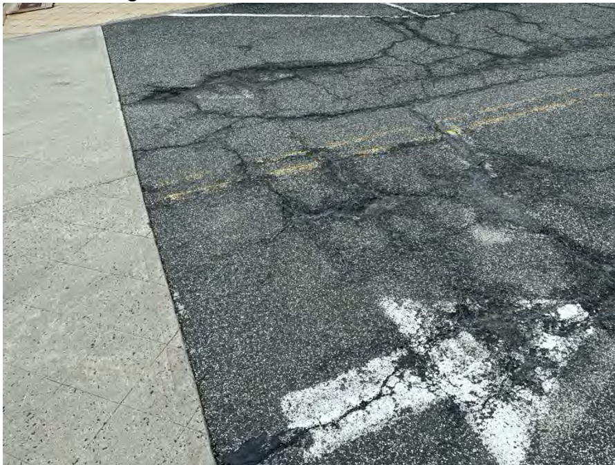
Figure 13: This entrance also has weathered striping to the point where the exit directional arrow is missing. To the uninitiated, this can seem be a one-way entrance to the lot, creating the potential for a motorist to not consider oncoming traffic exiting the lot.
