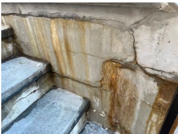
Figure 33: Weathered plastering around the foundation wall and base of the rear entrance stairs.
