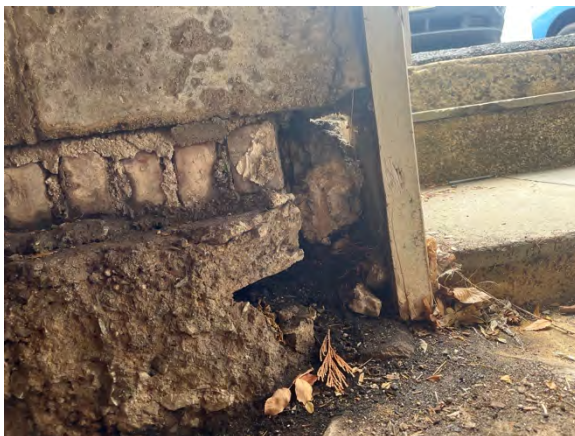
Figure 35: An example of an opening in the foundation wall of 5 Morristown Road.
