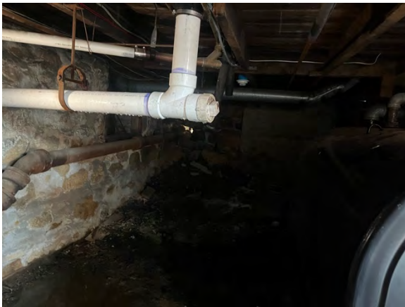
Figure 34: Leak in basement and standing water below.
