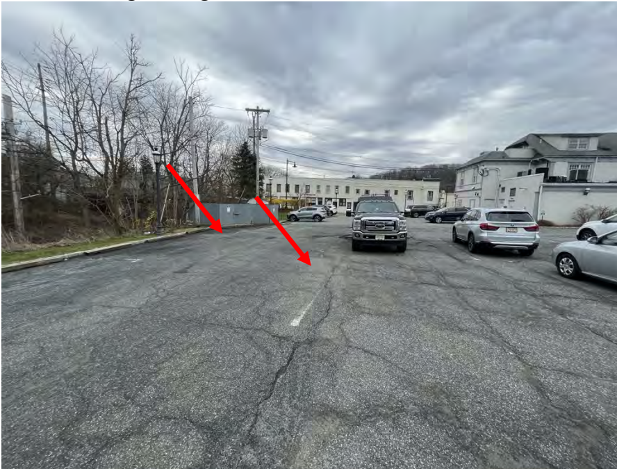
Figure 9: The curbing depicted on the southern portion of the site plan is missing. Features like this curbing are to guide the pattern of circulation on site and to protect parked vehicles from turning vehicles in motion. They also serve as an elevated surface for pedestrians, increasing their visibility to operators of moving vehicles and providing safe areas. With this curbing left out, neither of these purposes are being fulfilled. This is a condition detrimental to health and safety.
