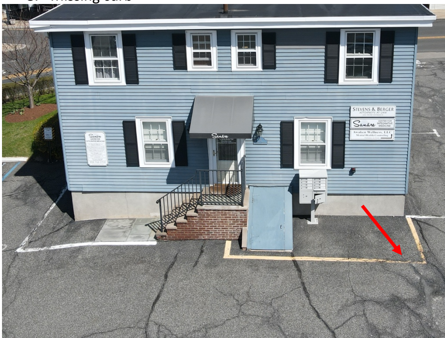
Figure 14: There is a curb missing at the base of the rear of 35 Olcott Square, which is indicated on the approved site plans. This deprives pedestrians of an elevated surface to make themselves more visible and allows for vehicles to make this turn more closely. This creates a point of conflict detrimental to health and safety. It also brings the base of the cellar door entry to the basement to the same height as the parking lot. This can cause issues of water seeping into the basement that could have been avoided if the curb was present.
