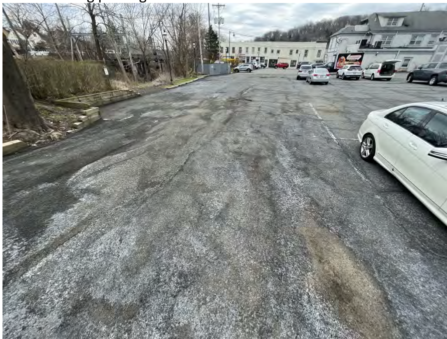
Figure 30: As mentioned above, several parking spaces are missing here that were indicated on the site plan. Consequently, this space is being utilized as an unapproved drive aisle for which no striping or directional arrows exist. This is another point of potential conflict between motorists and pedestrians, as the lack of any coherent marker of intended circulation is missing.
