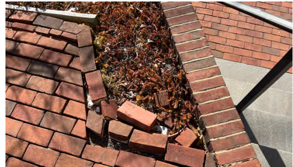
Figure 19: Bricks from paved pathway uneven and out of place
