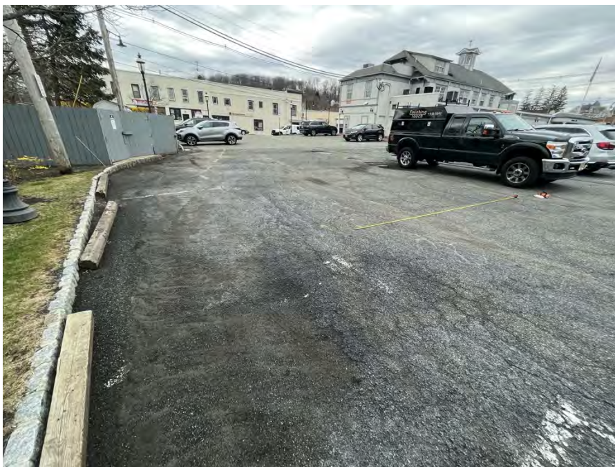
Figure 8: The parking in question narrows the drive aisle to under 16 feet wide. This unapproved parking reduces the functionality of the drive aisle which, despite the lack of corresponding striping, is intended to function to accommodate two-way traffic.
