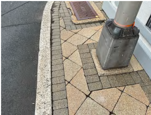
Figure 23: View of sidewalk along a section of Lot 1 with a utility pole obstructing use. The usable width is reduced to 25 inches; not enough space for a person using a wheelchair. An example of a seemingly small hurdle for a person with the ability to walk unimpeded by a disability affecting their capability to do so, this issue becomes insurmountable without substantial risk to a person who is wheelchair-bound. Such considerations are crucial for people with disabilities navigating spaces, especially public spaces such as this pedestrian right of way.
