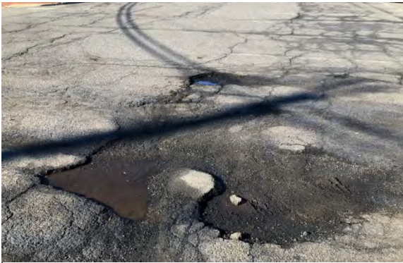
Figure 20: Cracked pavement and potholes
