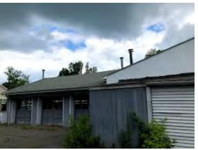
Figure 12: Peeling and blistered paint; deteriorating wood exteriors.
