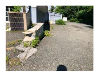
Figure 22: Damaged retaining wall.
