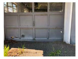
Figure 16: Cracked areas on and around door frames.
