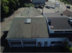
Figure 11: Aerial imagery suggests roof leakage.
