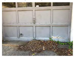
Figure 23: Accumulation of debris suggests draining issue.
