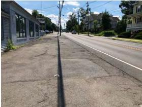
Figure 25: Cracked pavement.
