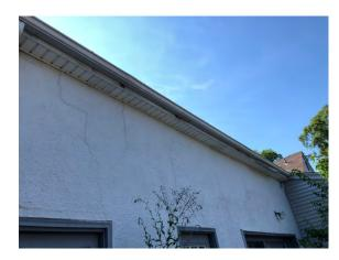
Figure 13: Cracks in stucco suggest developing structural issue.
